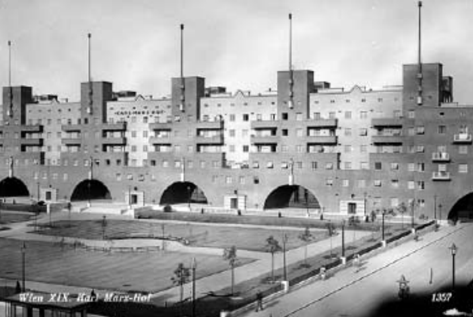
KARL-MARX-HOF. VIEW FROM AN ELEVATED POSITION TOWARD HEILIGENSTÄDTERSTRASSE
